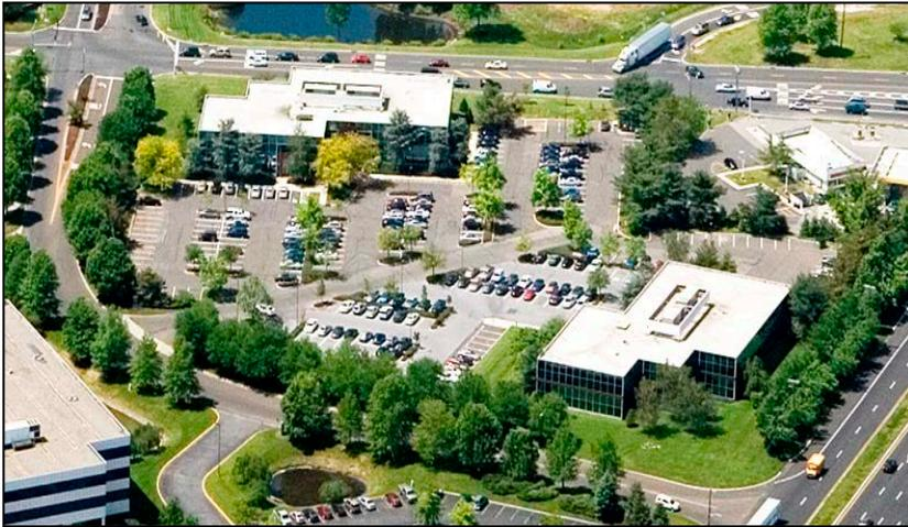
**Roof:** New TPO roofs were recently installed at each building. The white roofs reduce solar heat gain due to their reflective qualities which subsequently increases HVAC energy efficiency.
